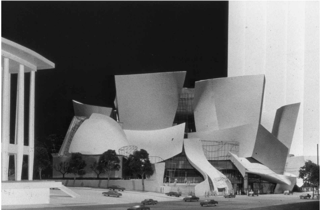
Figure 16. Walt Disney Concert Hall, Los Angeles, California, project model, photograph, Joshua White, Courtesy of Gehry Partners, LLP.
